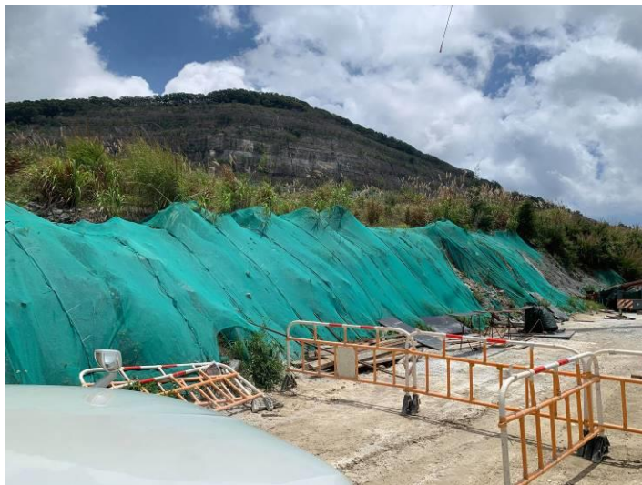
Impermeable cover for slope at System A.
