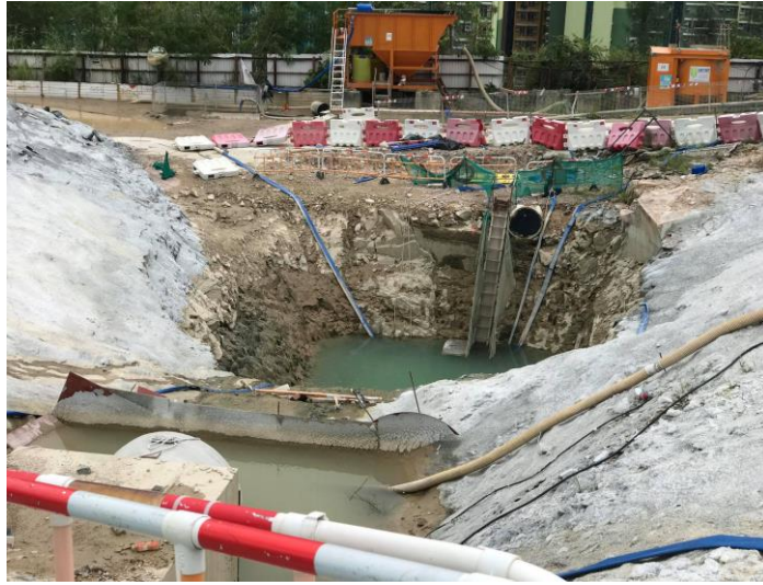
Paving for exposed slope to reduce dust dispersion & mitigate the silty runoff generation at Q1.
