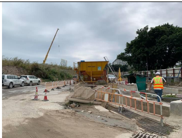
Q6: Wastewater treatment facility 24 cu. m.
