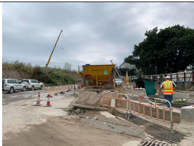
Q6: Wastewater treatment facility 24 cu. m.
