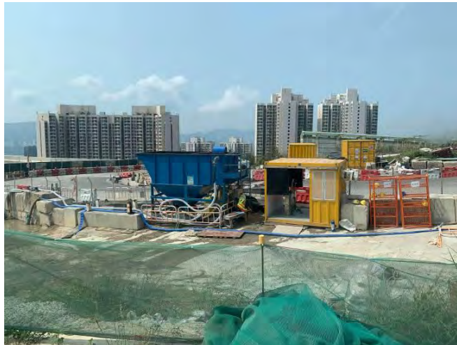
Q4. Wastewater treatment facility Temporary Water Reservoir 150 cu.m + AquaSed of 60 cu.m per hour
