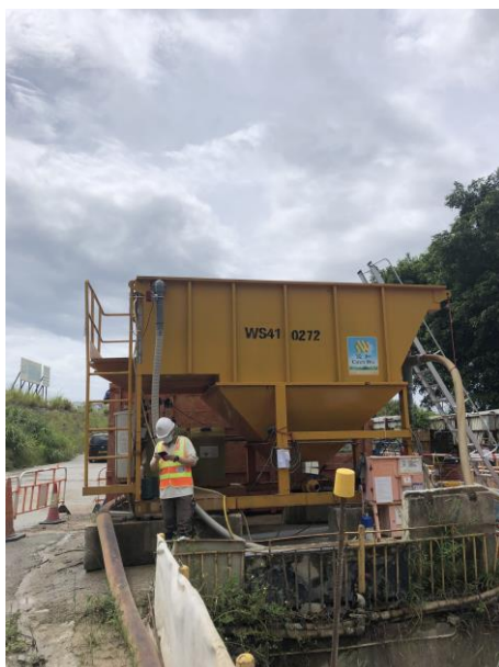
Q6: Wastewater treatment facility 24 cu. m.
