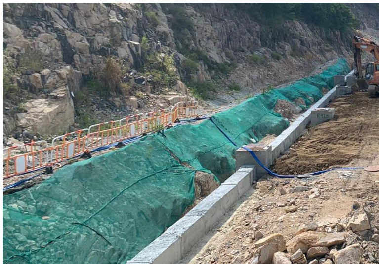
Impermeable cover for slope at PTT
