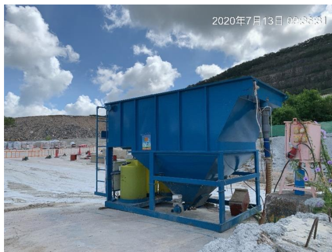
Q4. Wastewater treatment facility Temporary Water Reservoir 150 cu.m + AquaSed of 60 cu.m per hour
