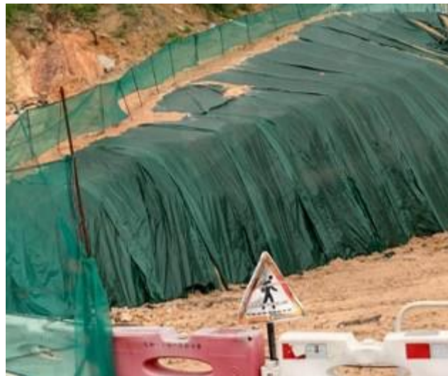
Impermeable cover for slope at Pumping Station
