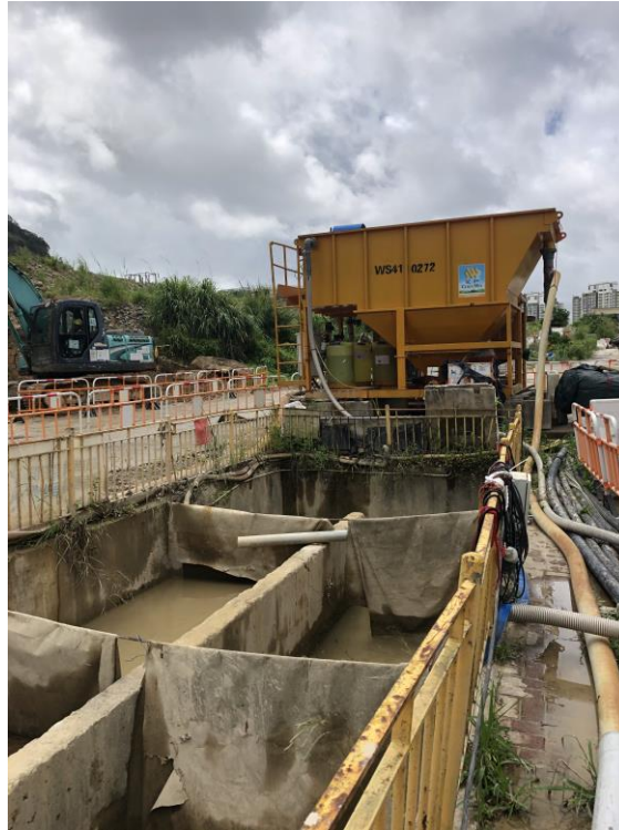
Q6: Wastewater treatment facility 24 cu. m.
