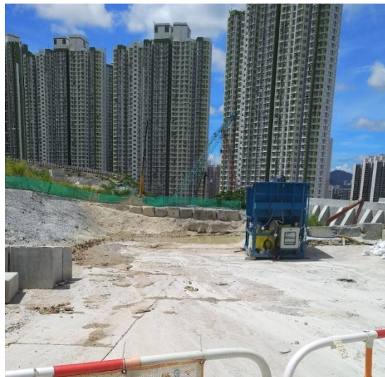
Q1. Wastewater treatment facility 30 cu.m Sedimentation Tank + AquaSed of 15 cu.m per hour
