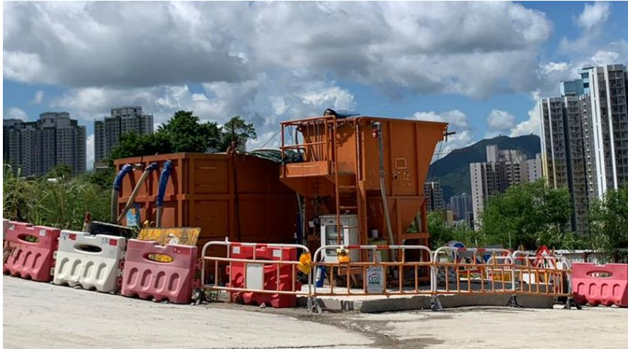
Q1. Wastewater treatment facility 30 cu.m Sedimentation Tank + AquaSed of 15 cu.m per hour
