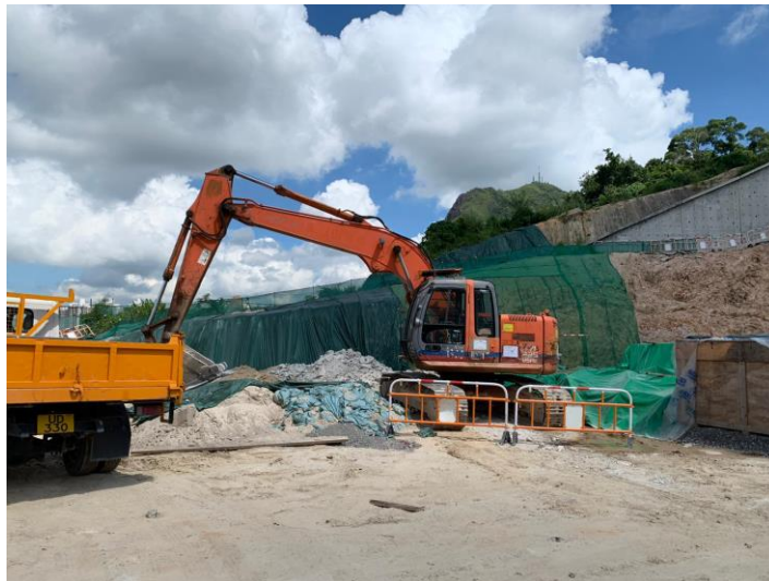
Impermeable cover for slope at Pumping Station
