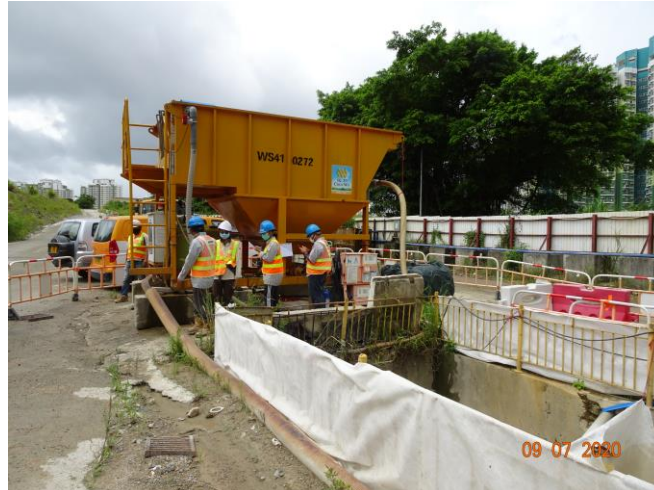
Q6: Wastewater treatment facility 24 cu. m.
