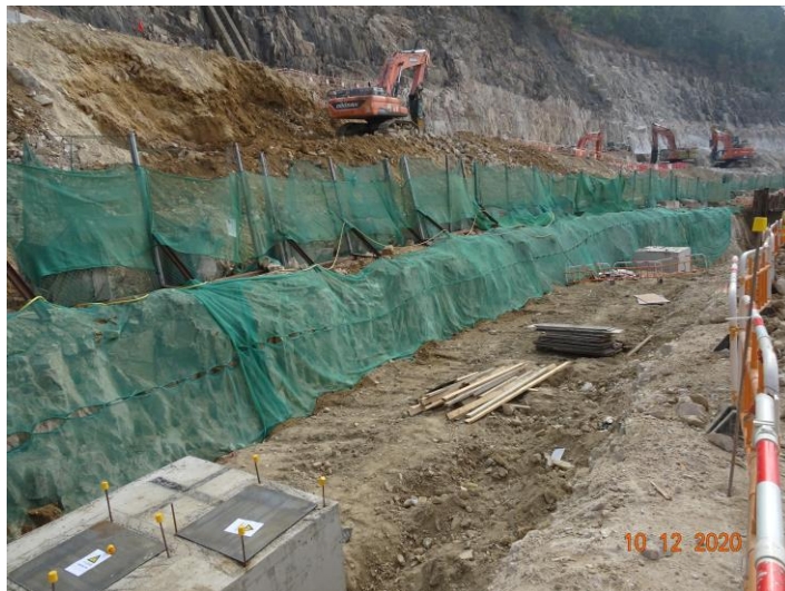
Impermeable cover for slope at PTT.
