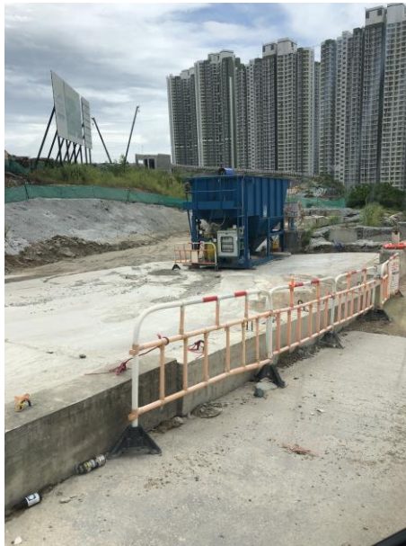
Q4. Wastewater treatment facility Temporary Water Reservoir 150 cu.m + AquaSed of 60 cu.m per hour
