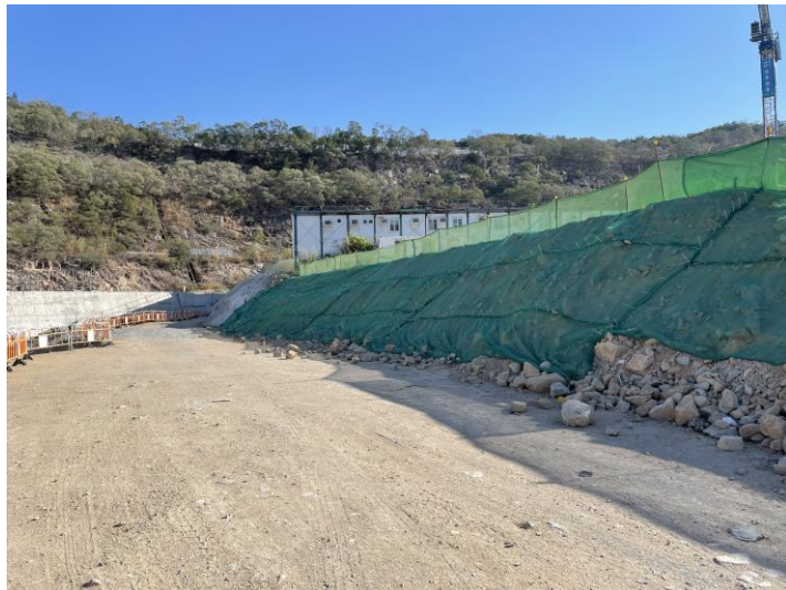
Impermeable cover for slope at Pumping station.
