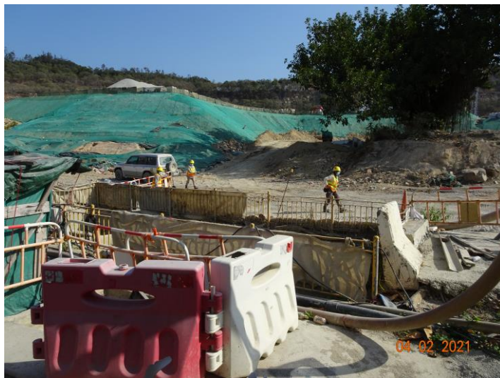
Impermeable cover for slope at Q5.
