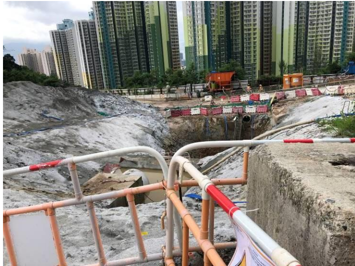
Paving for exposed slope to reduce dust dispersion & mitigate the silty runoff generation at Q1.
