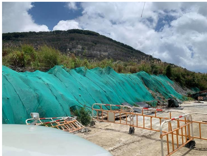
Impermeable cover for slope at System A.
