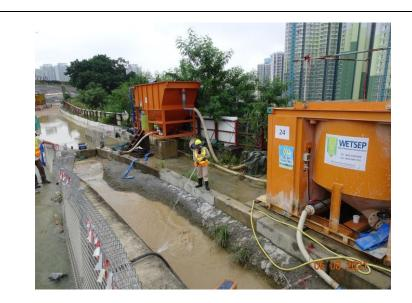
Q1. Wastewater treatment facility 30 cu.m Sedimentation Tank + AquaSed of 15 cu.m per hour + WETSEP
