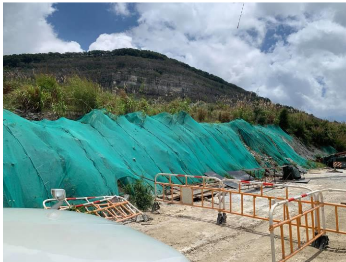
Impermeable cover for slope at System A.
