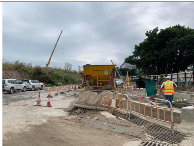
Q6: Wastewater treatment facility 24 cu. m.
