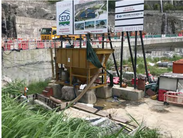
Q7. Wastewater treatment facility 30 cu.m Sedimentation Tank + AquaSed of 60 cu.m per hour
