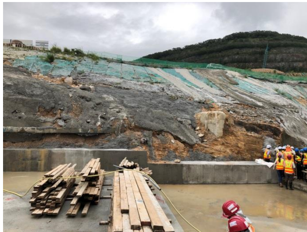
Exposed surface was covered by cement mortar
