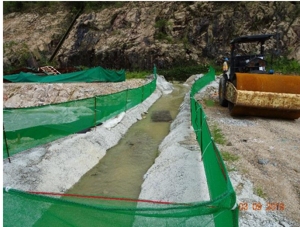
Perimeter channel to collect site surface
