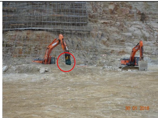
Photo 3 As noise mitigation measures, the head of the breakers were wrapped by acoustic materials.
