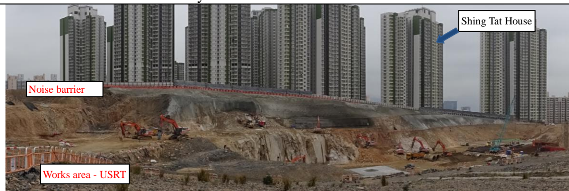
Photo 2 Excavation and breaking works were carried out at USRT and there was direct line of sight between the construction site and the upper floor of Shing Tat House. As noise mitigation measures, erection of acoustic mat as temporary noise barrier was installed along the boundary of Portion A toward On Tat Estate
