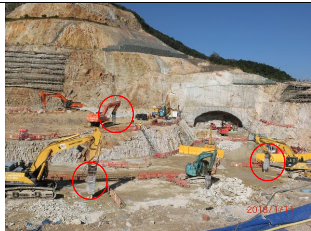
Photo 4 As noise mitigation measures, the head of the breakers were wrapped by acoustic materials.
